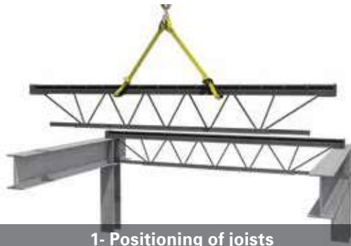
1- Positioning of joists
