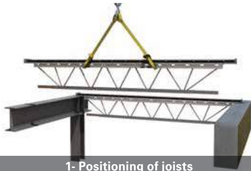
1- Positioning of joists
