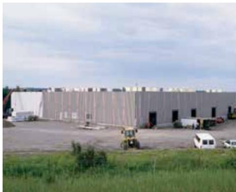
Erection of the steel structure and wall panels is completed. Once the steel deck is installed, the other sub-trades can start working.
